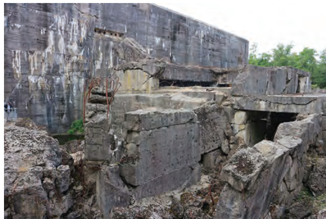
The north wall and in the foreground the shattered remains of the transit and servicing halls. Photo Bob Clary
